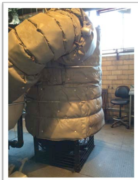
Figure 2.4 : Outer view of the gasifier
