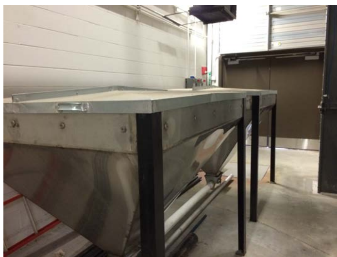
Figure 2.3 : Secondary Fuel Bin
